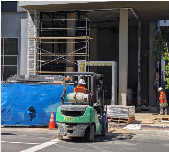
Construction of Inkwell, 2024
